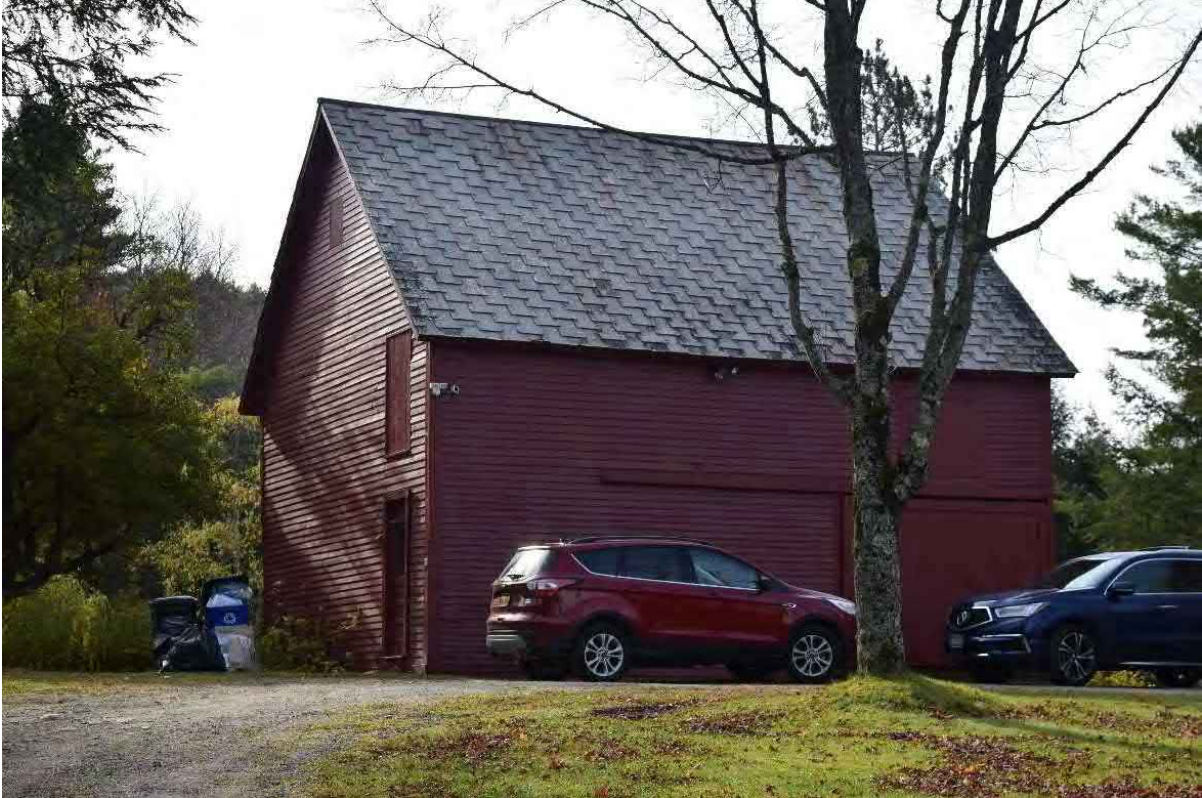
Photo 21. Barn associated with Structure 5, 691 Main Street, facing southwest.
