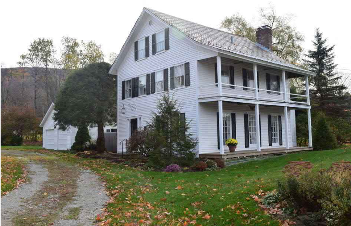
Photo 31. Structure 9, 3 Markham Lane, facing east.
