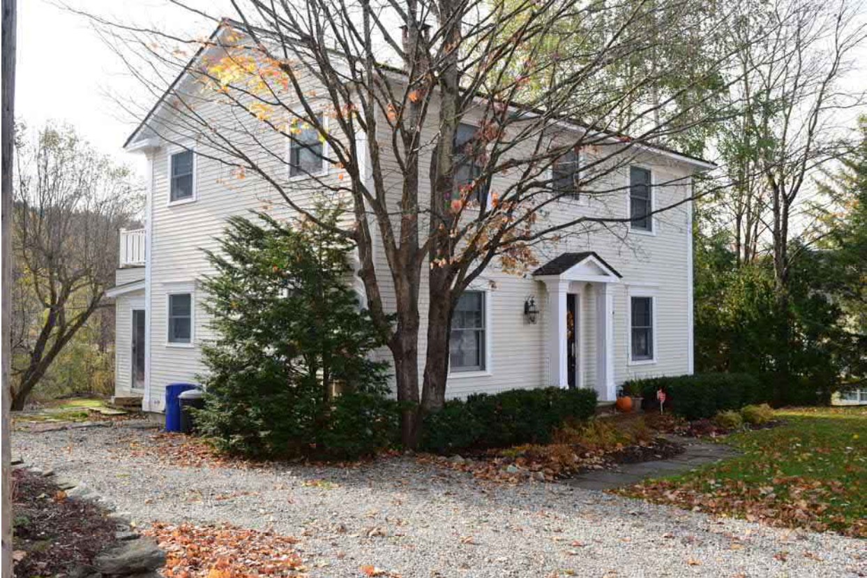
Photo 25. Structure 7, 685 Main Street, facing south.
