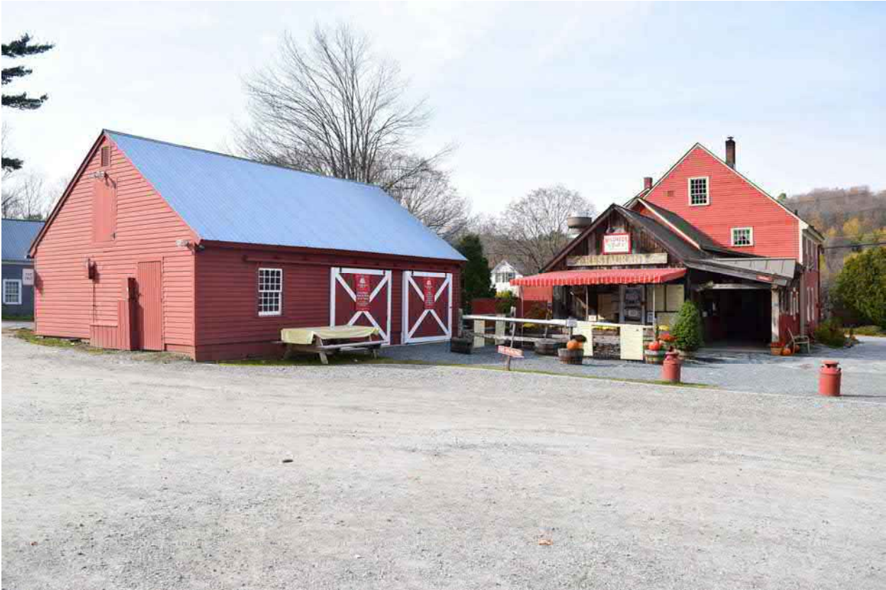
Photo 43. Rear view of 649 Main Street, facing southwest.
