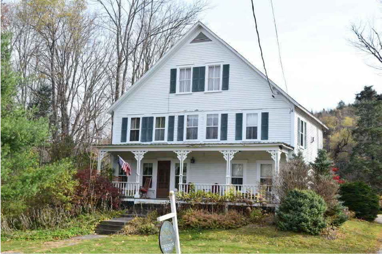
Photo 49. Structure 13, 633 Main Street, facing northeast.
