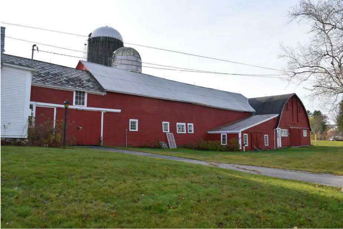
Photo 11. Shed/Barn wing and Hay/Cow Barn wing associated with Structure 2, facing southeast.
