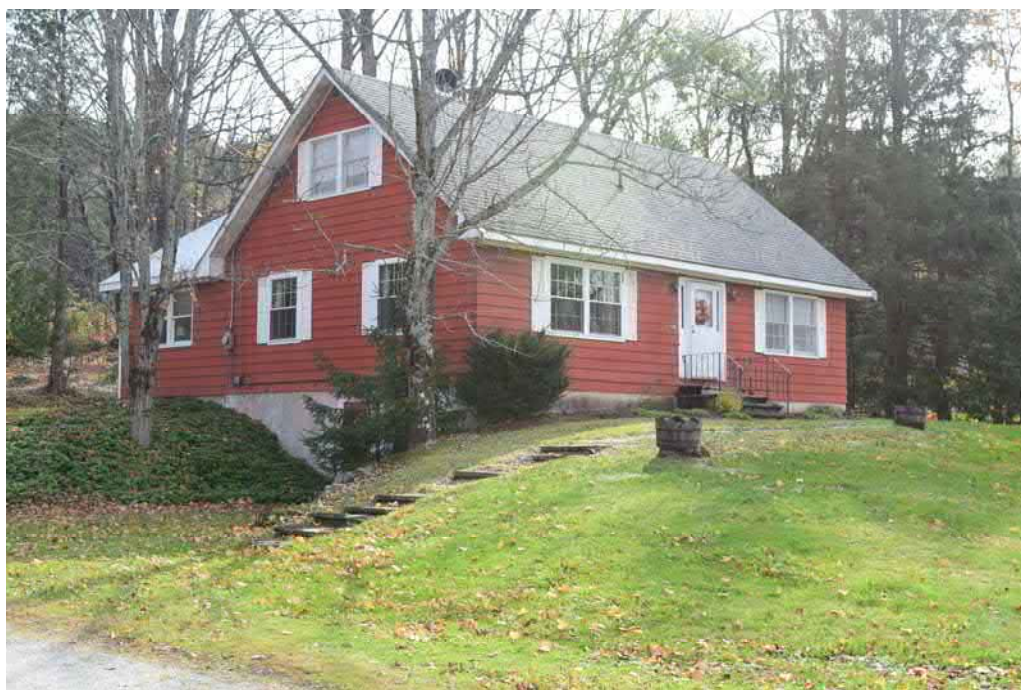
Photo 47. Structure 12, 639 Main Street, facing southeast.
