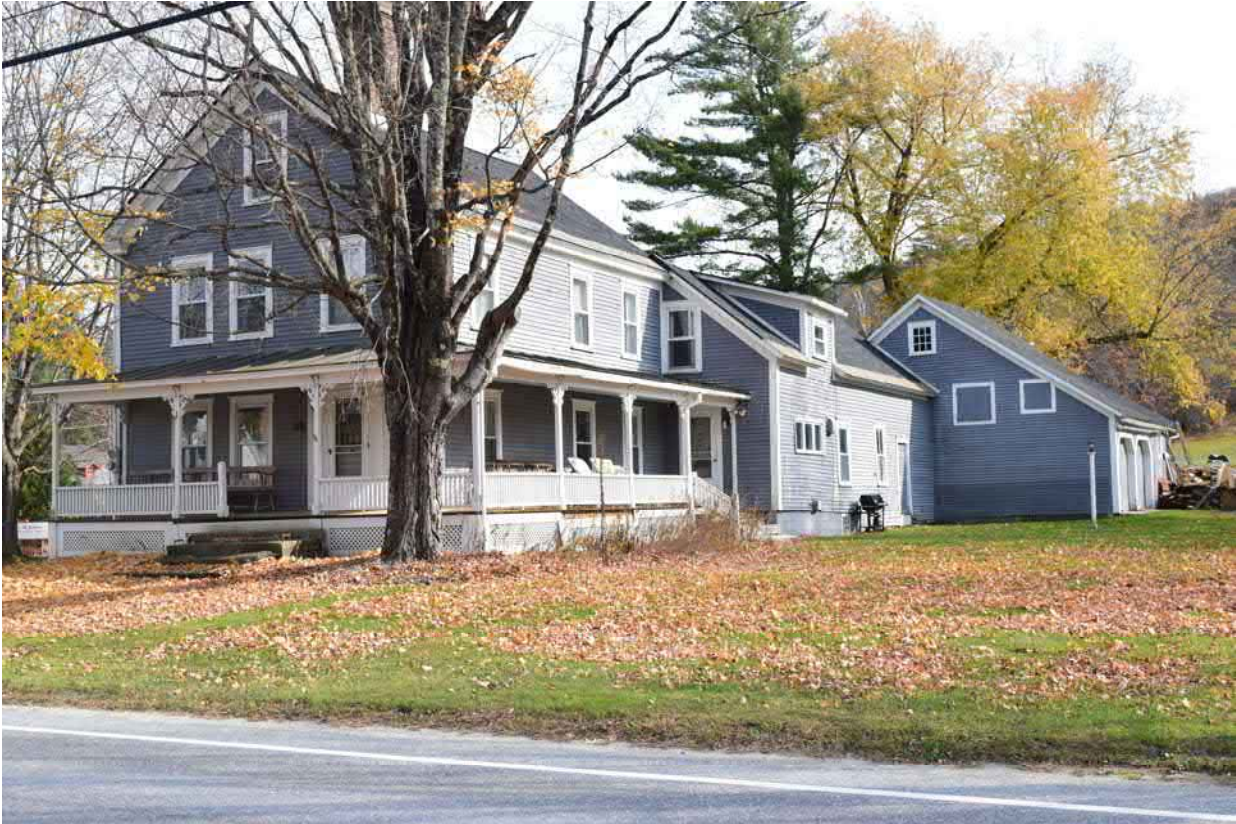
Photo 45. 647 Main Street, facing east.
