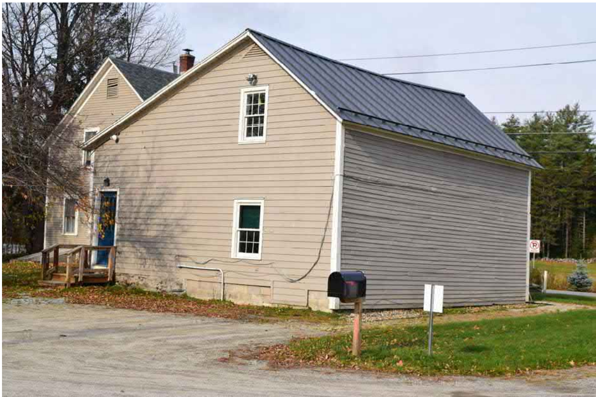
Photo 16. Structure 3, 703 Main Street, facing northwest.
