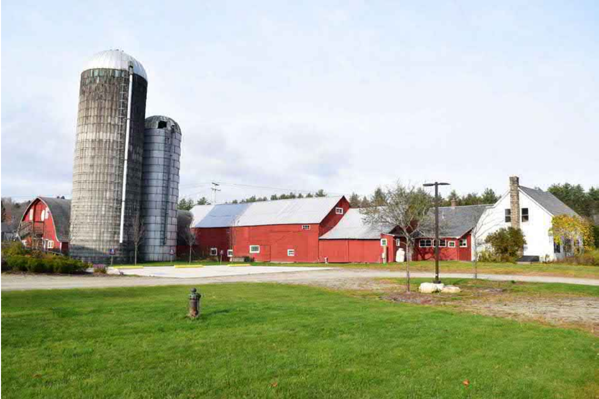
Photo 13. Rear view of Structure 2 at 725 Main Street, facing northwest.
