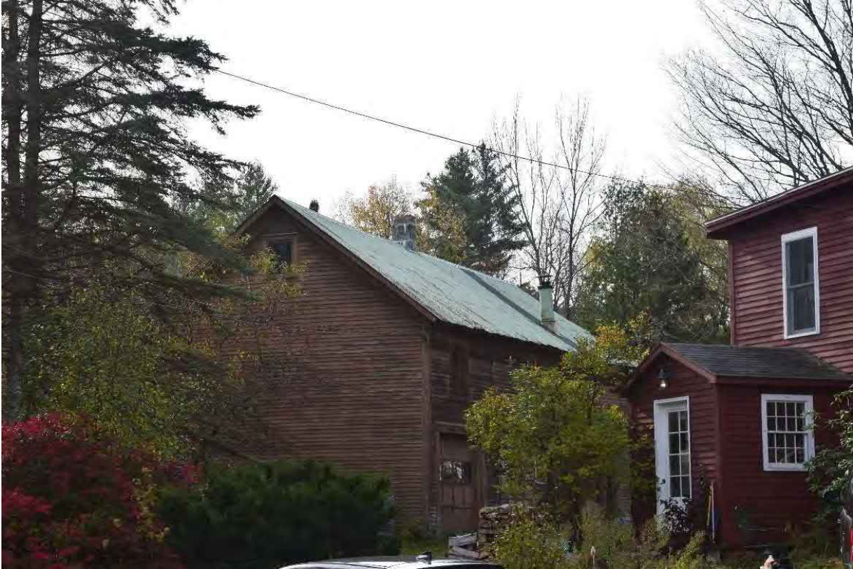
Photo 19. Structure 4, 699 Main Street, facing south.
