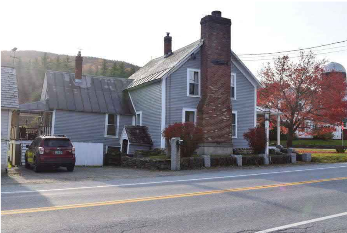
Photo 7. Structure 1, 725 Main Street, facing southeast.
