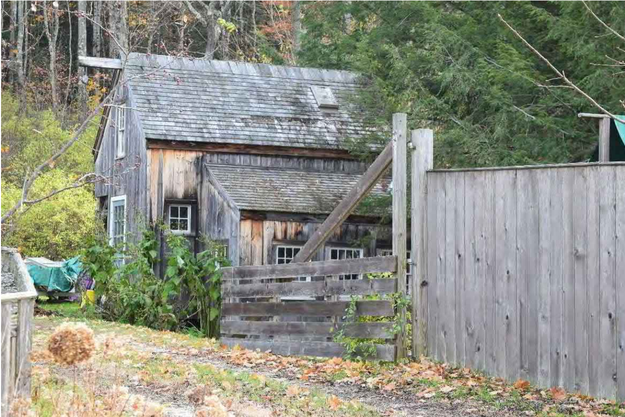
Photo 56. Outbuilding associated with Structure 16, facing east.
