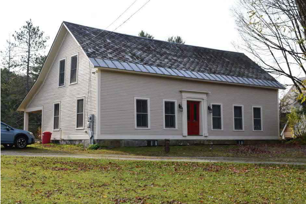
Photo 20. Structure 5, 691 Main Street, facing south.
