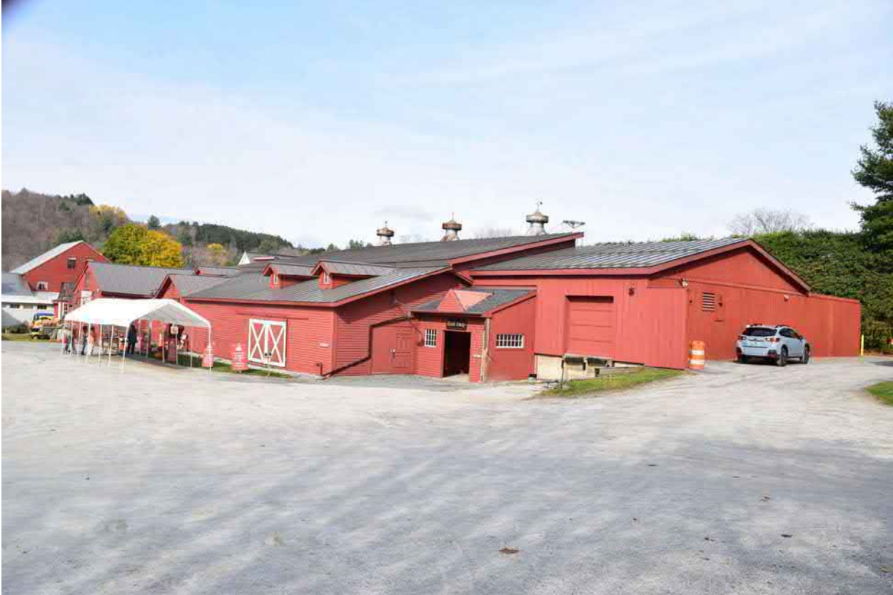
Photo 40. Rear view of 651-657 Main Street, facing northwest.
