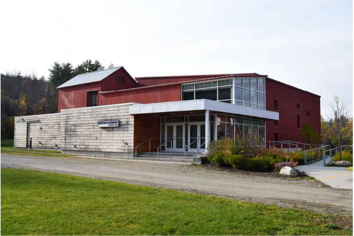
Photo 14. Weston Playhouse at Walker Farm, completed in 2017 on the property, facing southwest.
