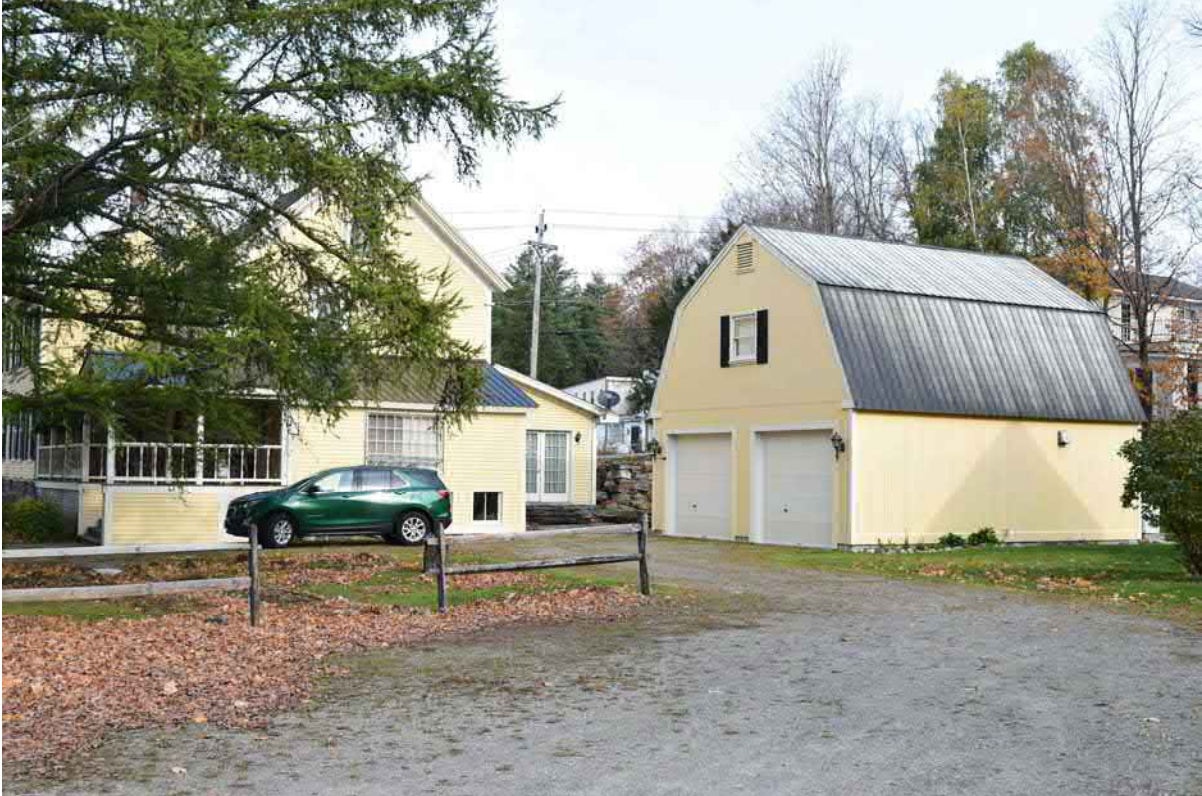
Photo 28. Structure 8, 4 Markham Lane, facing northwest.
