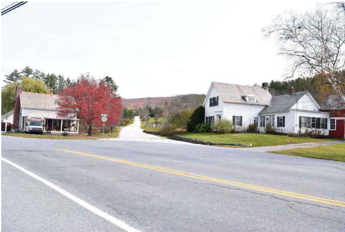
Photo 2. View of the intersection of Chester Mountain Road and Vermont State Route 100, facing northeast. Structures 1 and 2 in view.
