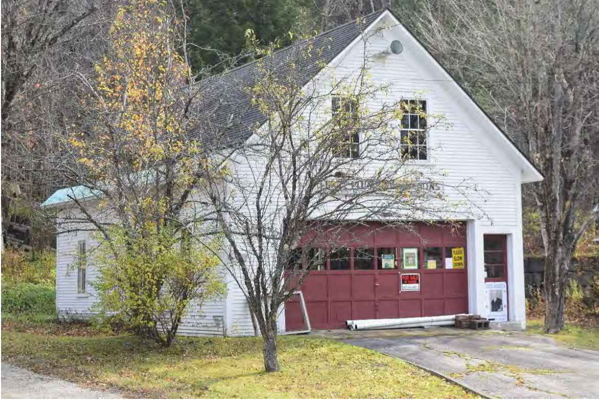
Photo 51. Structure 14, 629 Main Street, facing southeast.
