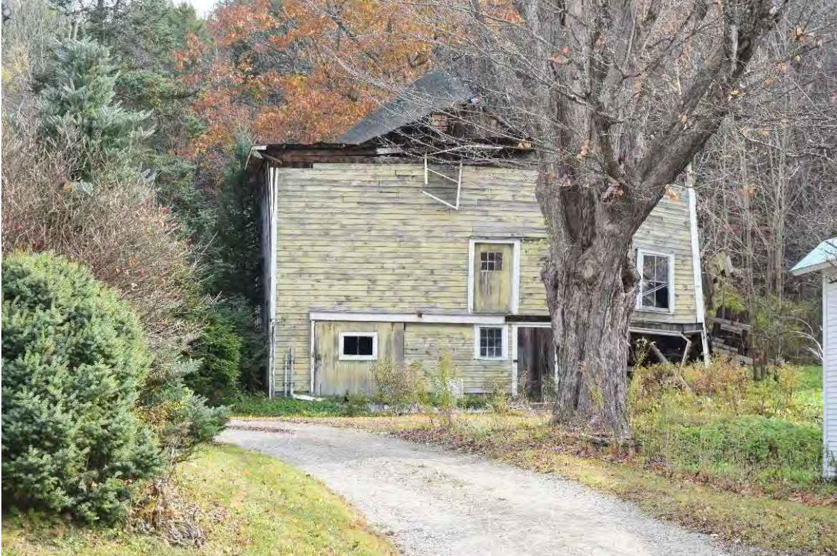
Photo 50. Barn associated with Structure 13, facing east.
