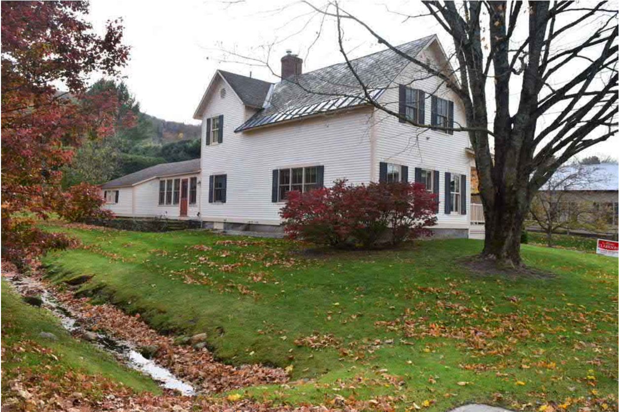
Photo 35. Structure 10, 665 Main Street, facing southeast.
