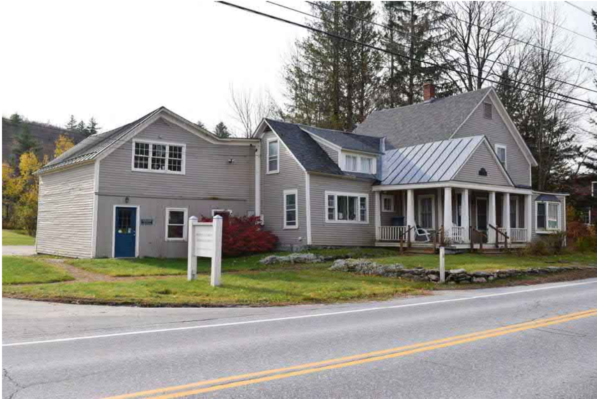
Photo 15. Structure 3, 703 Main Street, facing south.
