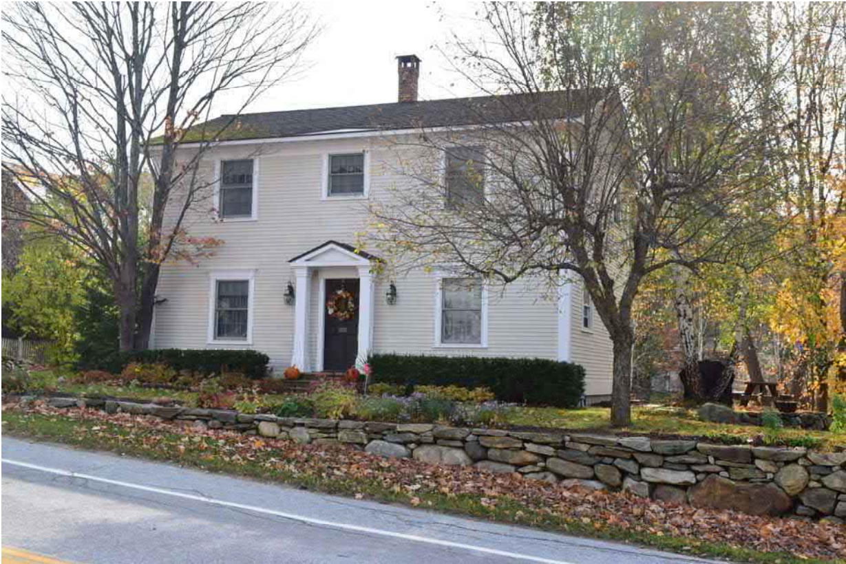
Photo 26. Structure 7, 685 Main Street, facing south
