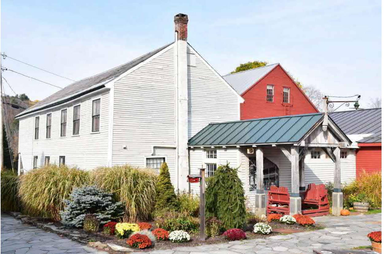
Photo 41. Rear view of 651-657 Main Street, facing northwest.
