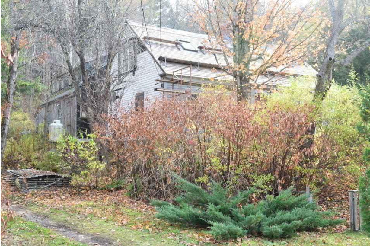
Photo 55. Structure 16, 623 Main Street, facing southeast.
