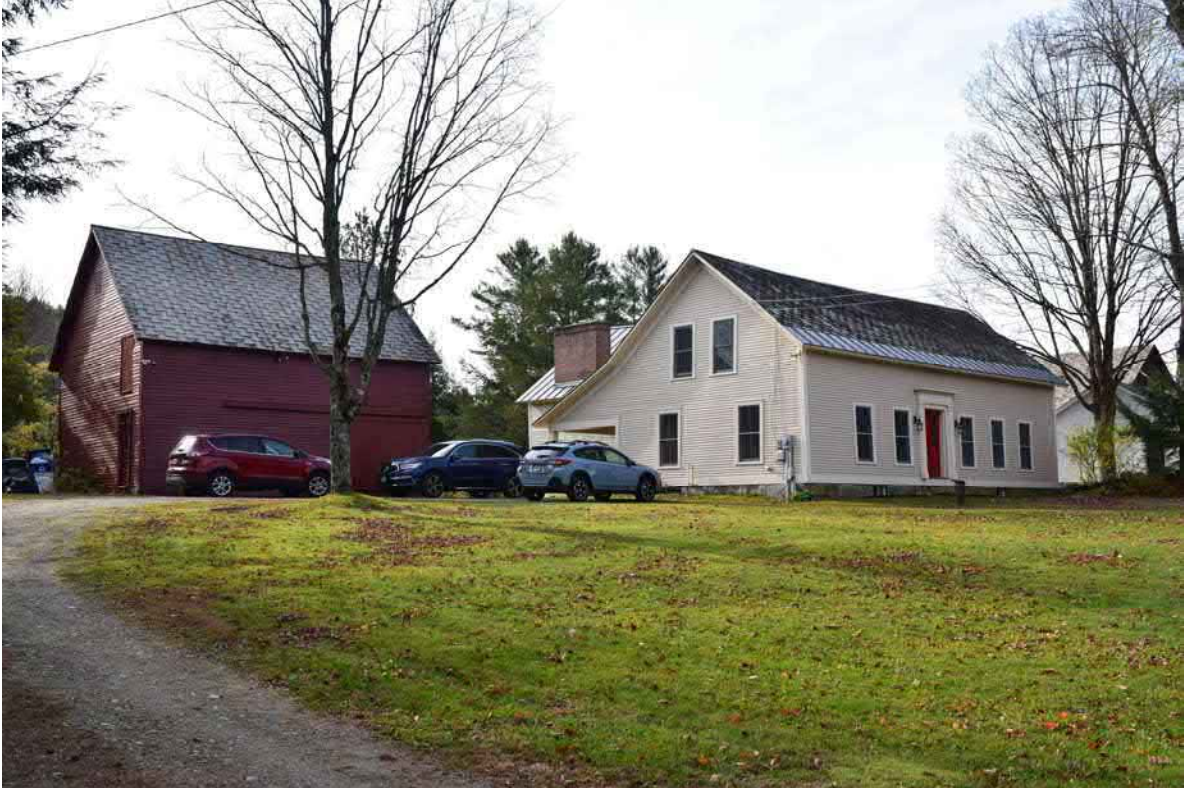
Photo 22. Structure 5, 691 Main Street, facing south.
