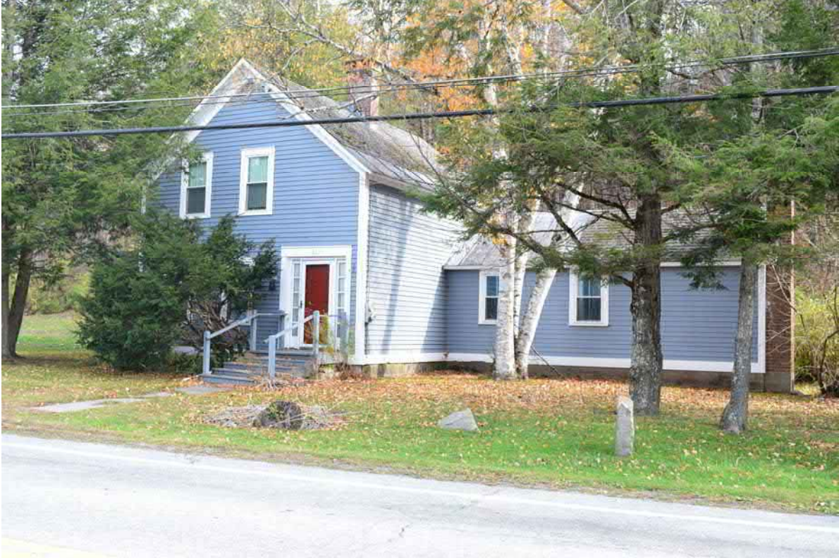
Photo 57. Structure 17, 613 Main Street, facing northeast. A granite hitching post seen in foreground at right.
