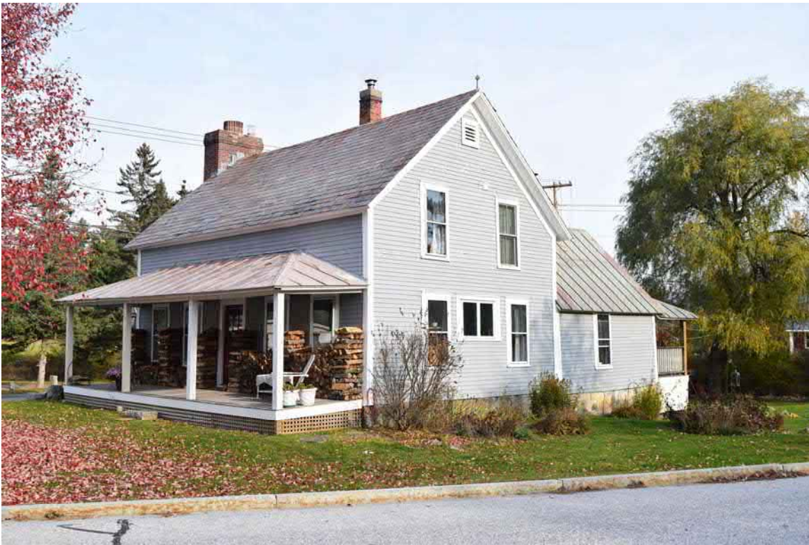
Photo 6. Structure 1, 725 Main Street, facing northwest.
