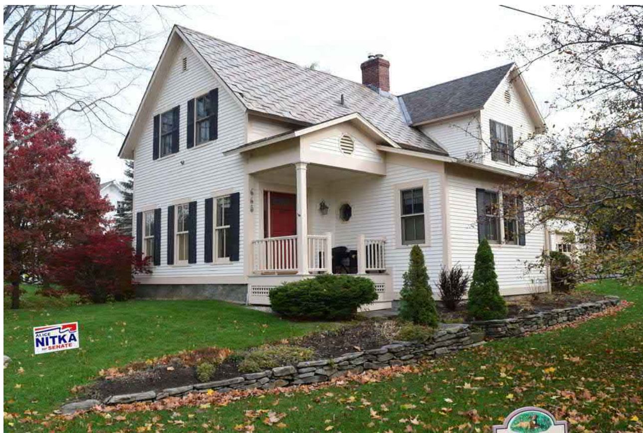
Photo 33. Structure 10, 665 Main Street, facing northeast.
