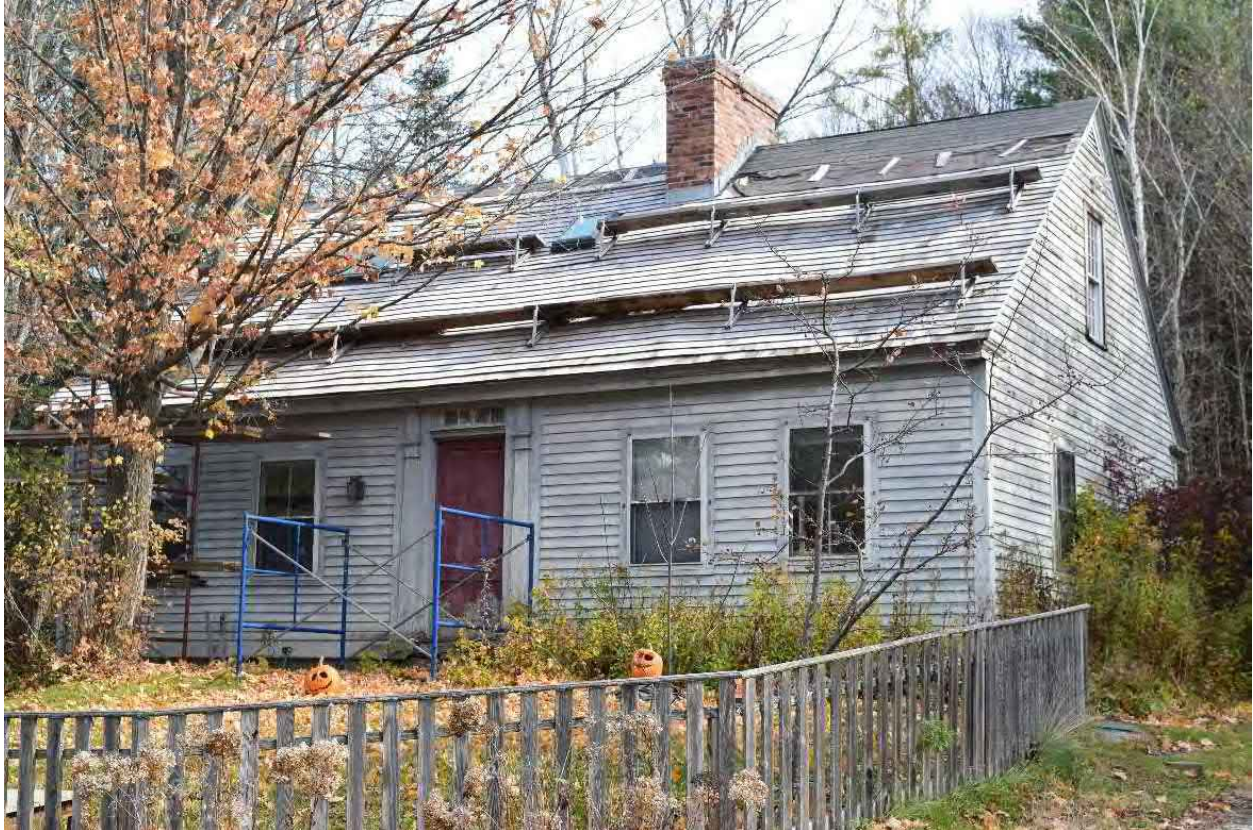
Photo 54. Structure 16, 623 Main Street, facing northeast.
