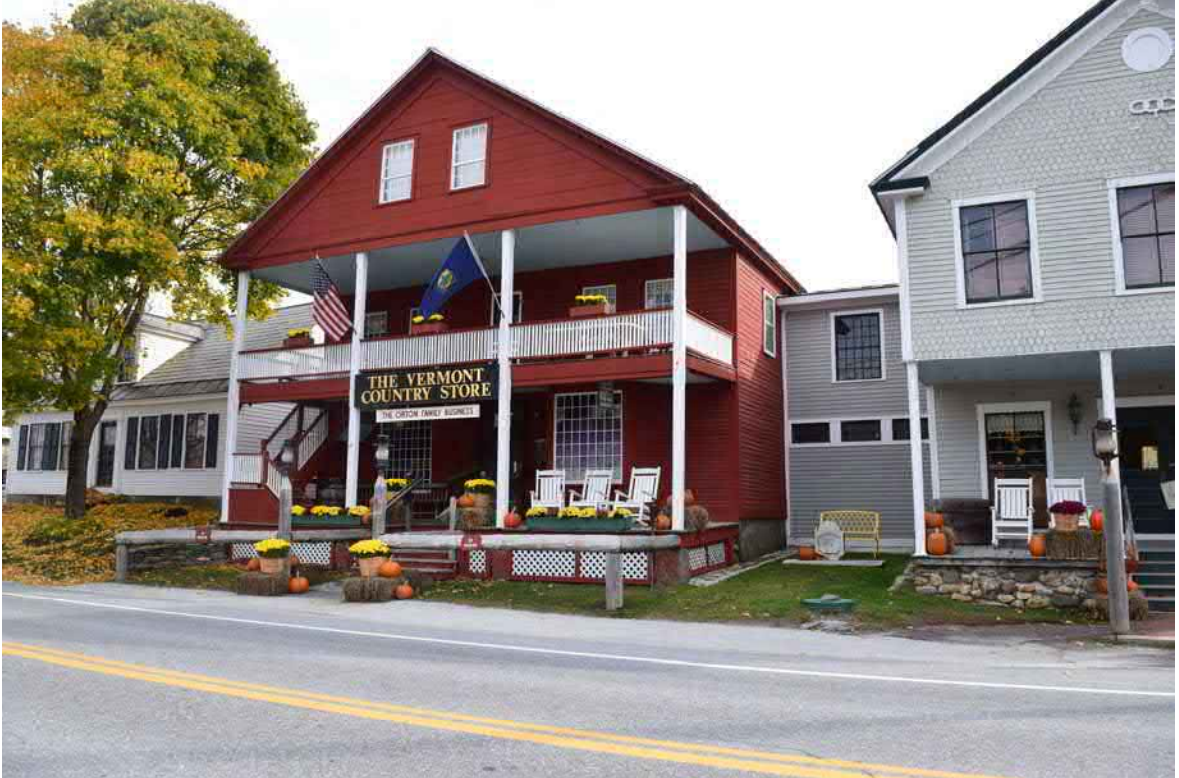
Photo 38. 651-657 Main Street, facing northeast.
