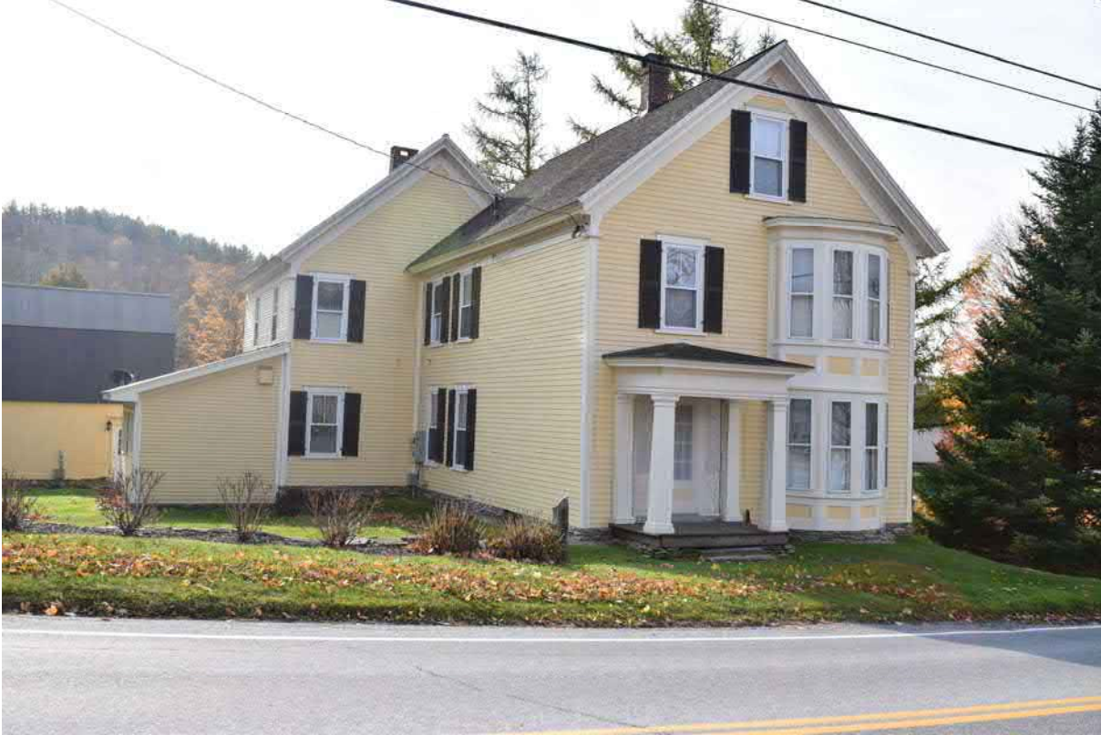
Photo 27. Structure 8, 4 Markham Lane, facing south.
