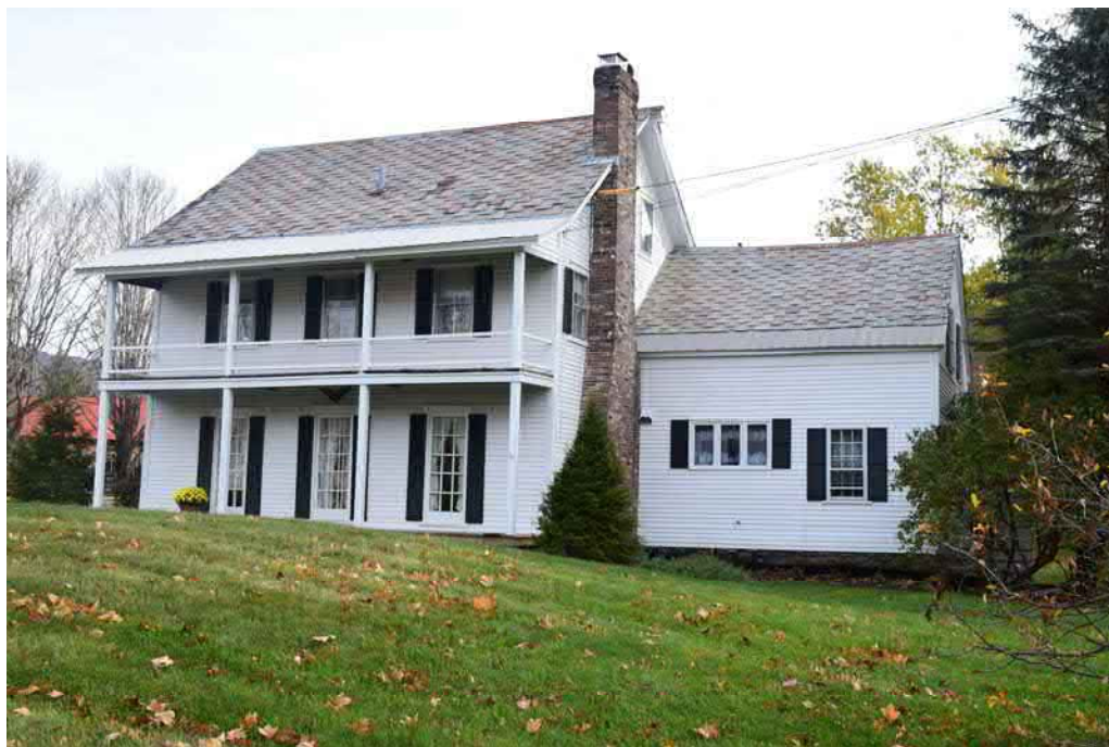
Photo 30. Structure 9, 3 Markham Lane, facing east.
