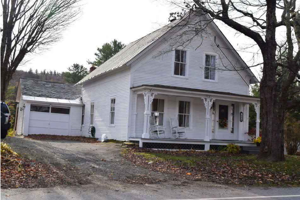
Photo 23. Structure 6, 689 Main Street, facing south.
