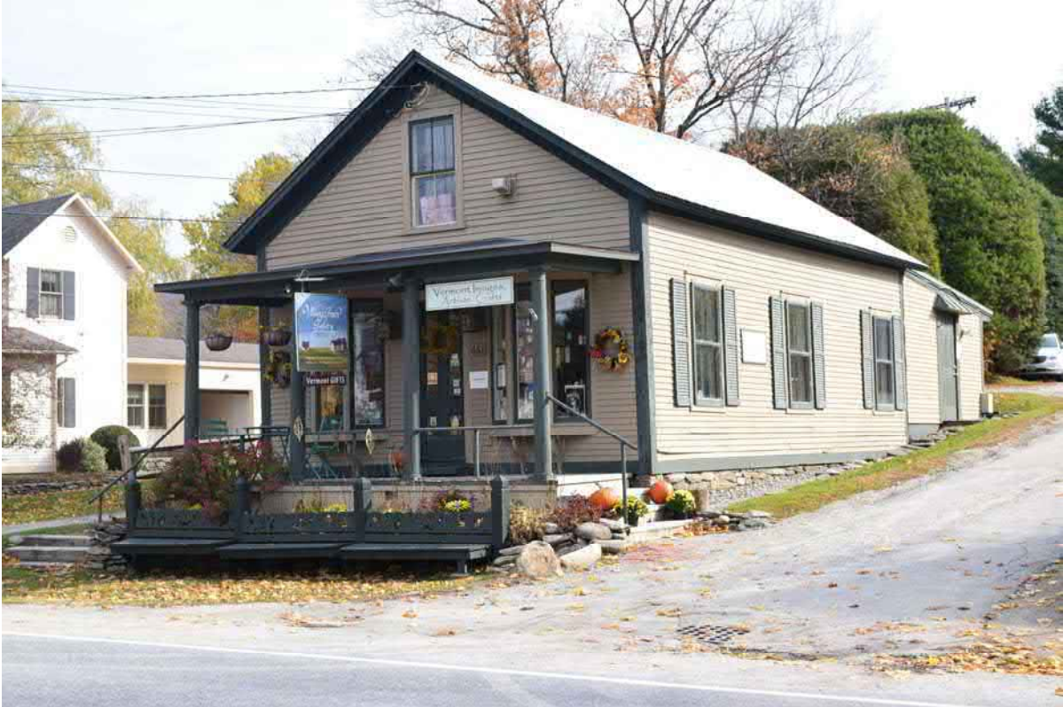
Photo 36. 661 Main Street, facing northeast.
