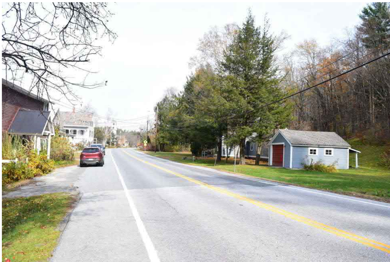
Photo 5. View looking north up Vermont Route 100. Structure 17 in view at right.
