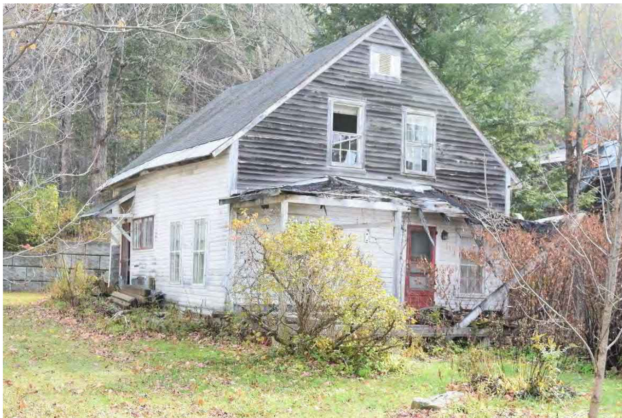
Photo 53. Structure 15, 627 Main Street, facing southeast.
