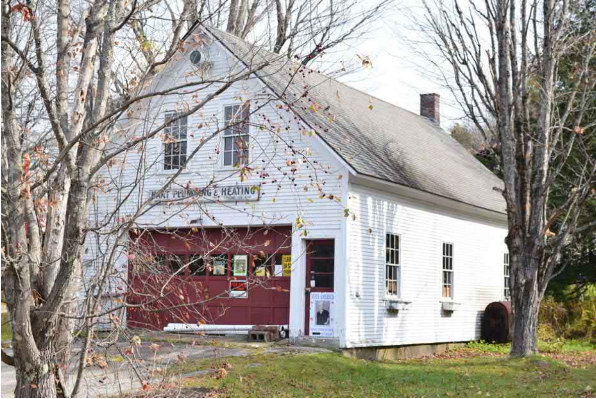
Photo 52. Structure 14, 629 Main Street, facing southwest.
