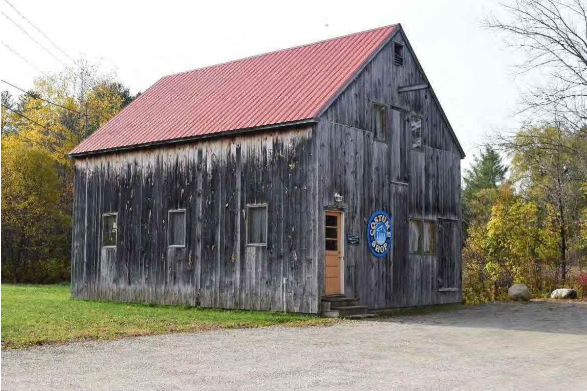
Photo 17. Outbuilding associated with Structure 3, facing south.
