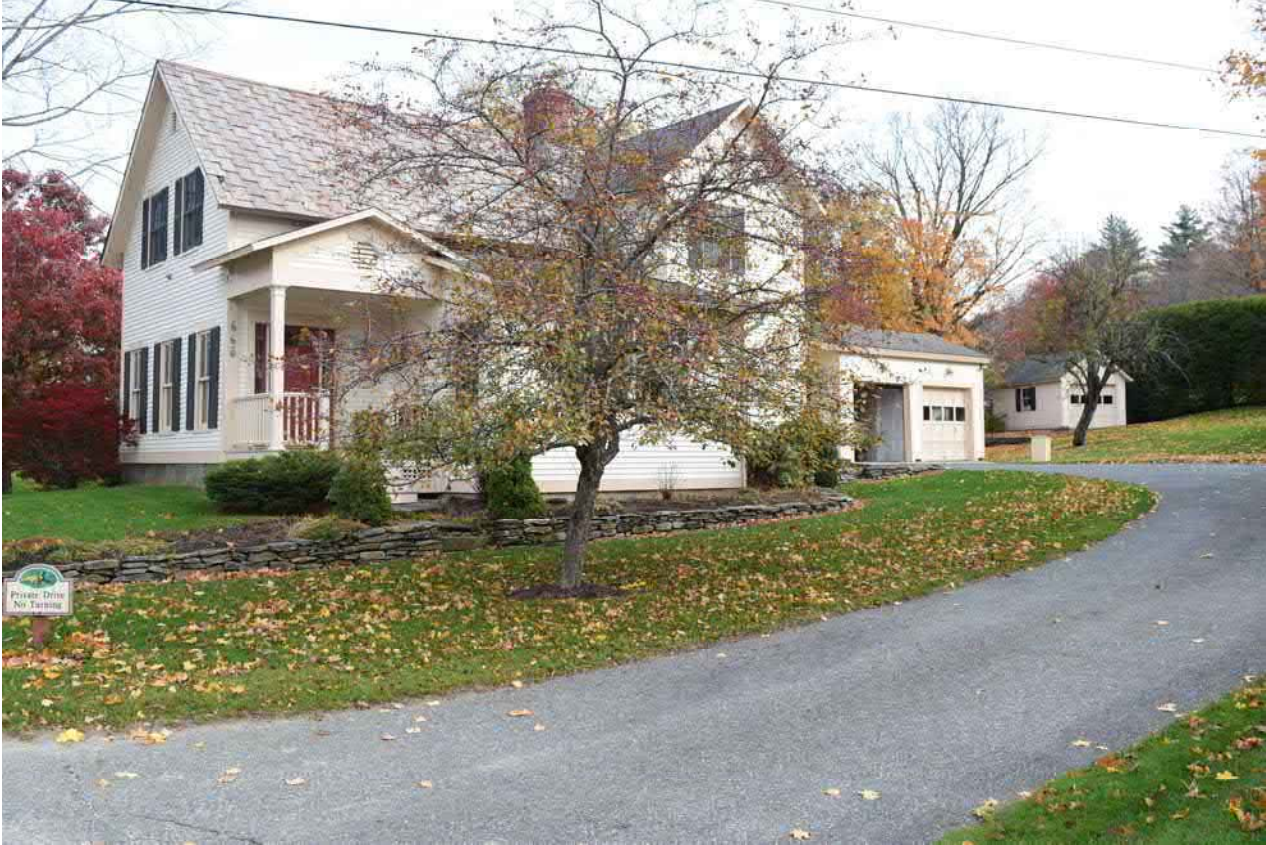
Photo 34. Structure 10, 665 Main Street, facing northeast.
