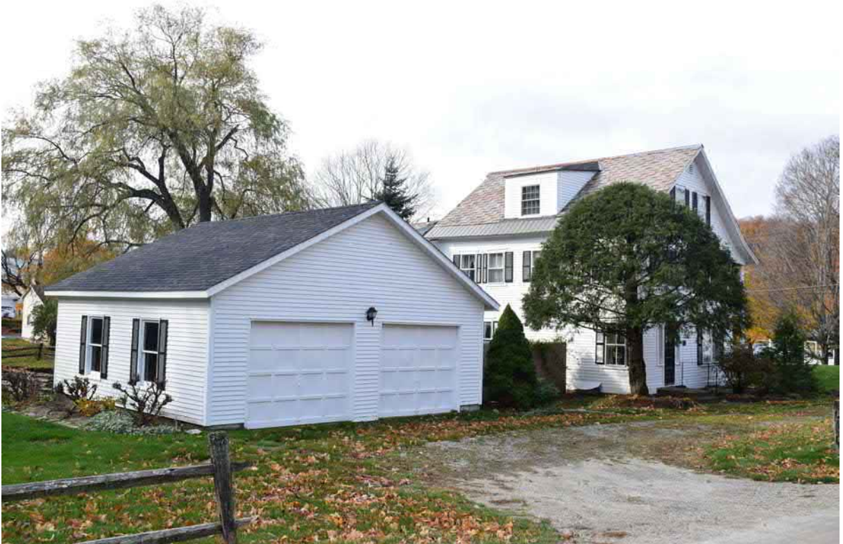
Photo 32. Structure 9, 3 Markham Lane, facing southwest.
