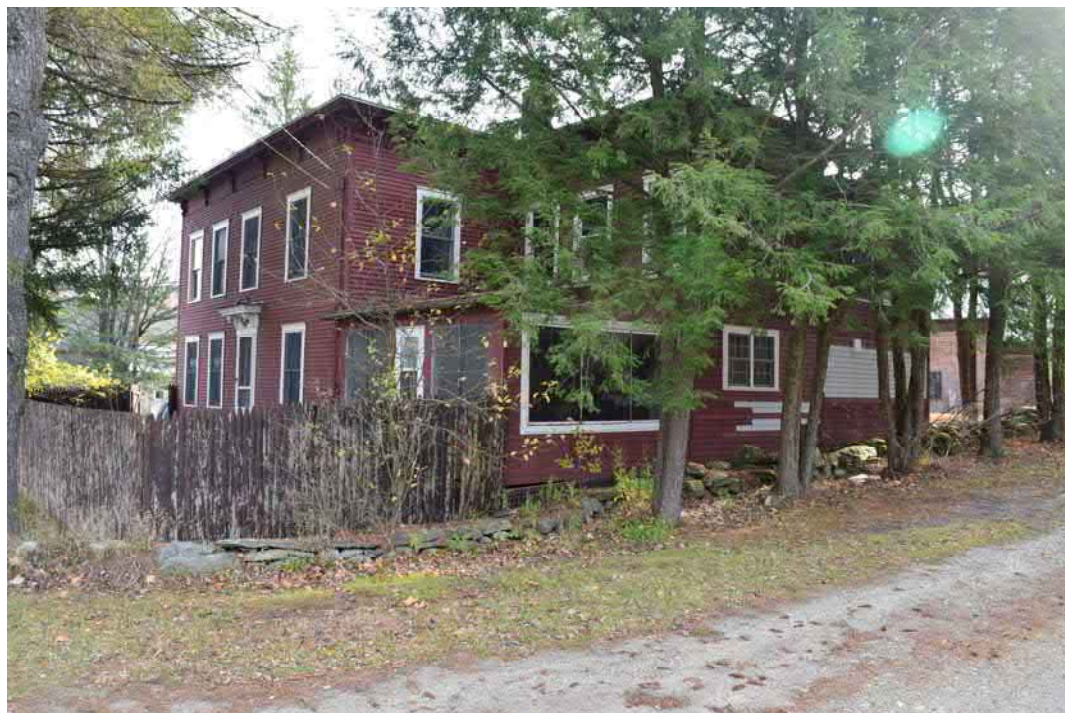
Photo 18. Structure 4, 697 Main Street, facing southeast.
