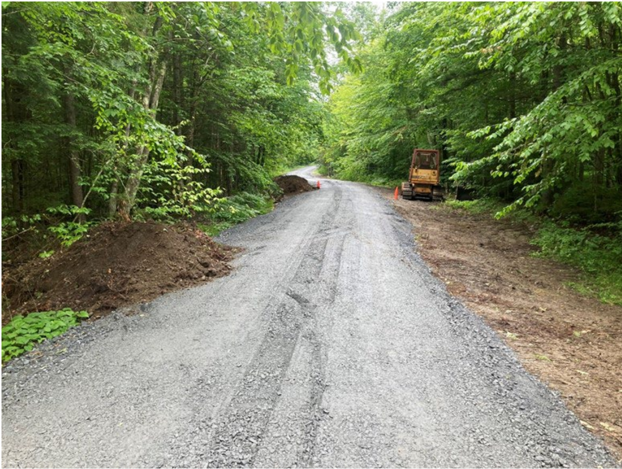
Photo 4 Construction work being done on the Forest Road 39 in Hancock. USDA Forest Service photo.
