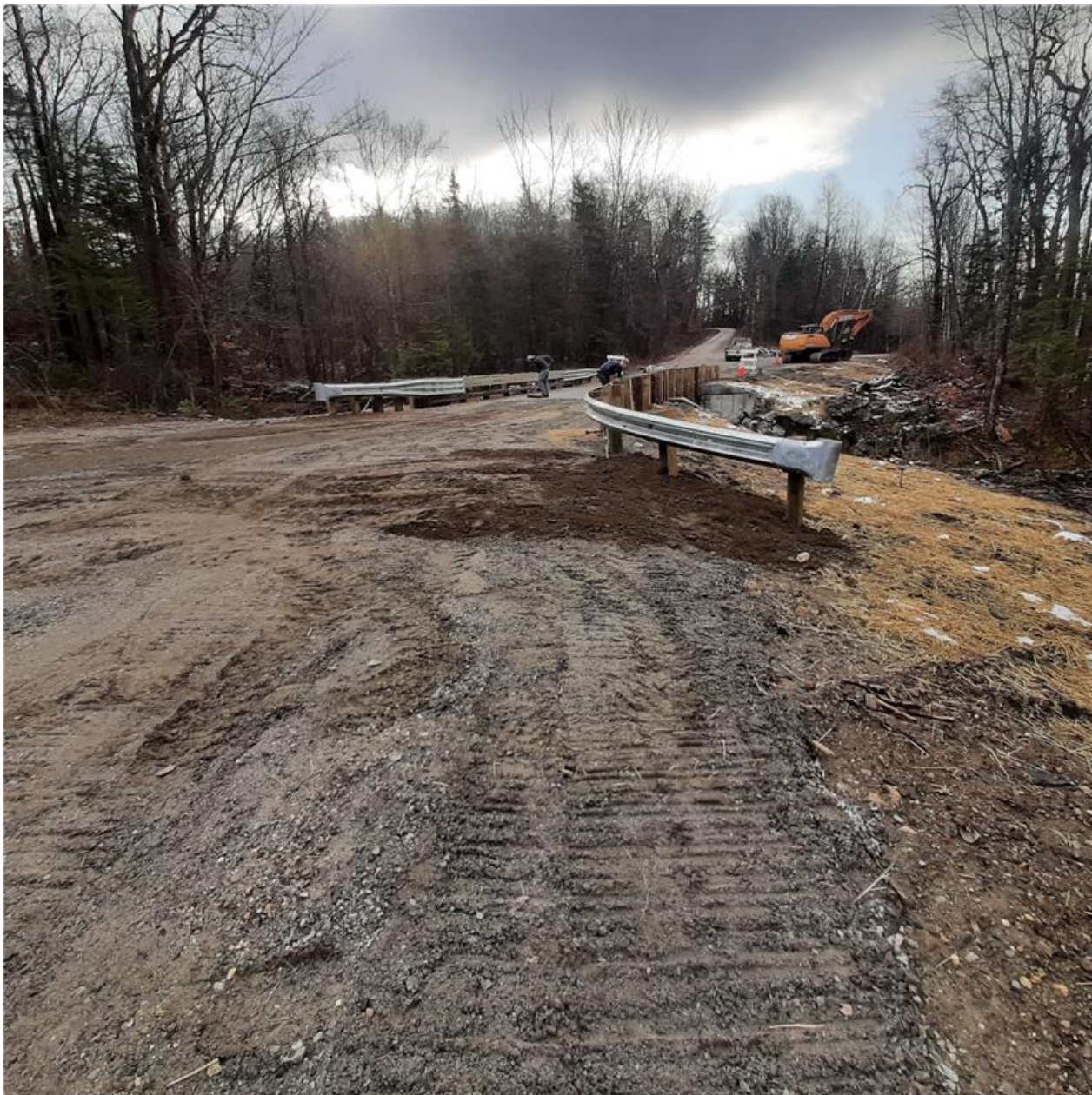
Photo 3 Construction work being done on the Forest.
